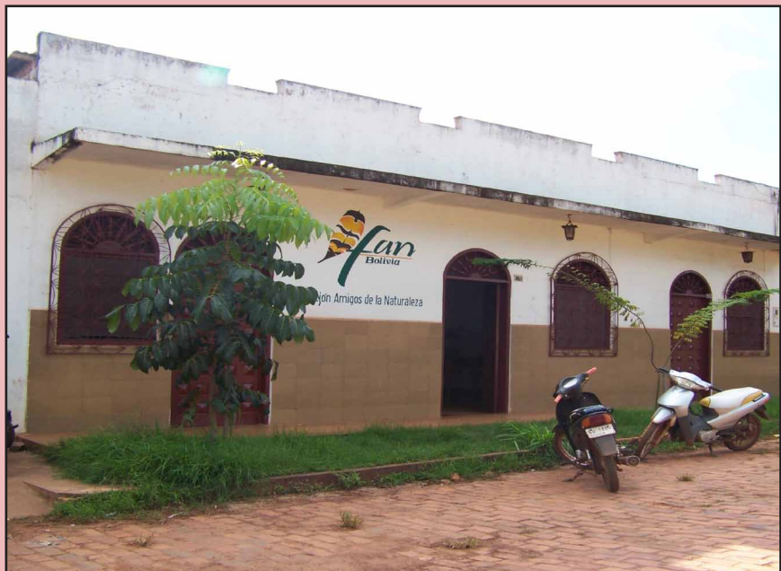
The offices of FAN, Riberalta - Kylie Benton-Connell
